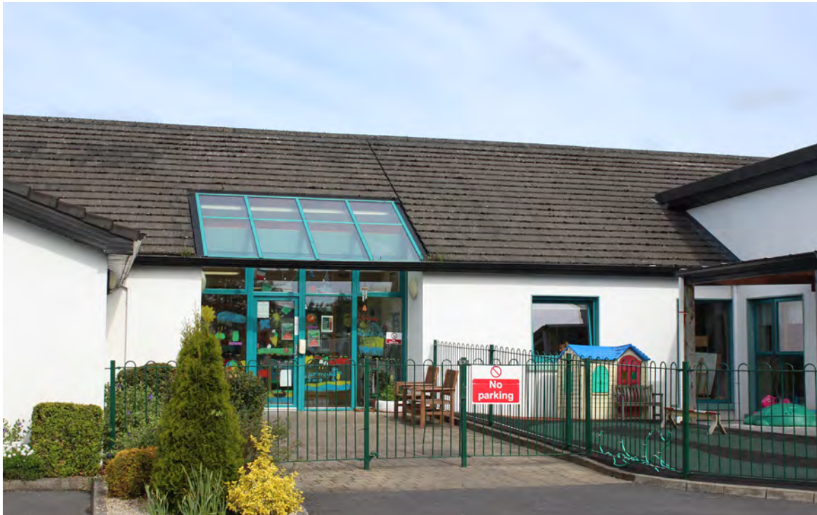
Figure 30. Entrance areas and main entrance doors to an ELC setting. Ballinderreen Community Childcare and Education, Ballinderreen, County Galway.
