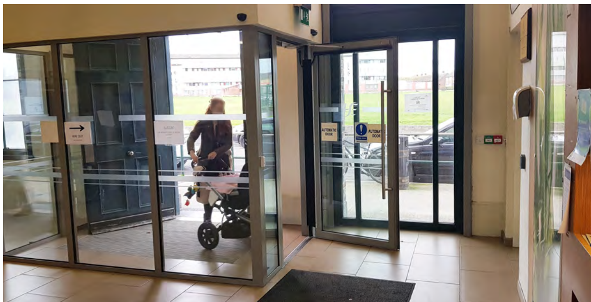
Figure 50. Power operated door providing easy access for person with buggy.
